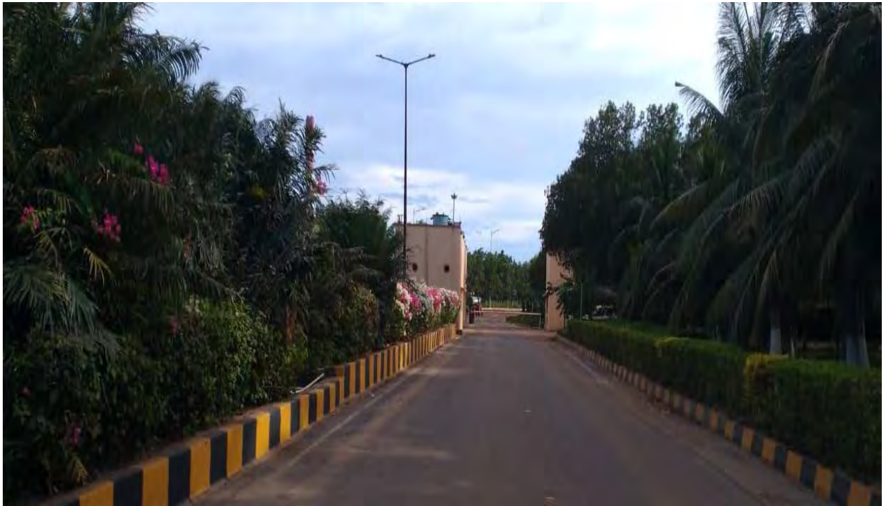
GREEN COVER NEAR PLANT SERVICE BUILDING
