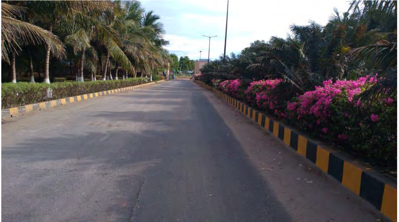
GREEN COVER ALONG PIPE RACK & INTERNAL ROADS
