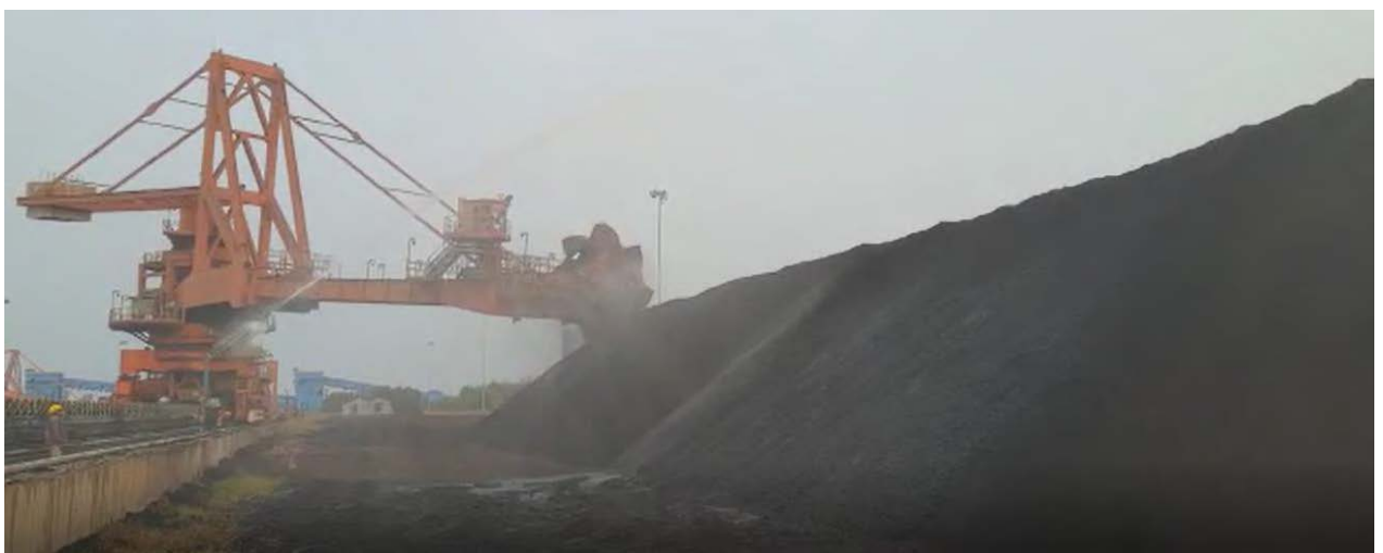
COAL YARD WATER SPRINKLING
