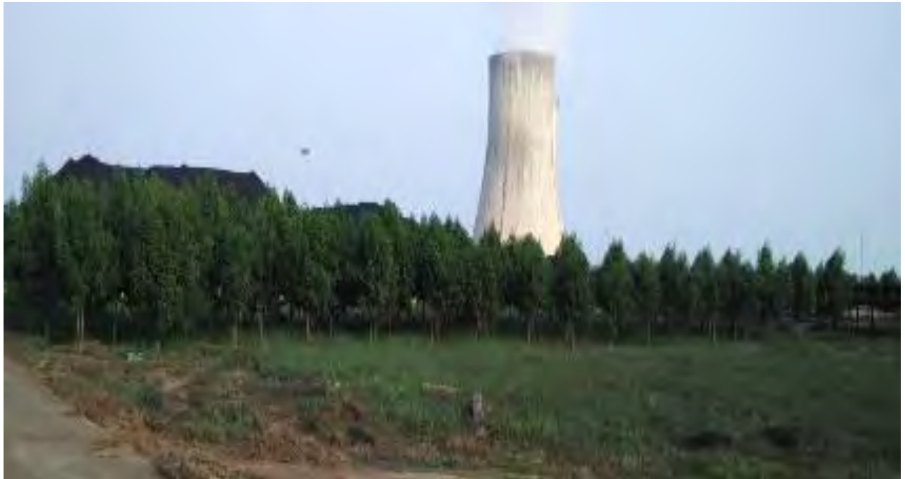
WIND BREAK PLANTATION AROUND COAL YARD
