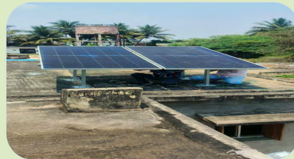
Off-grid solar on Anganwadi center
