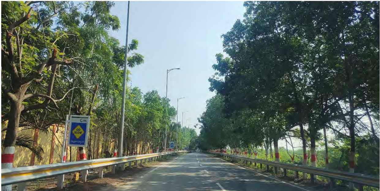
GREEN COVER ALONG PIPE RACK & INTERNAL ROADS
