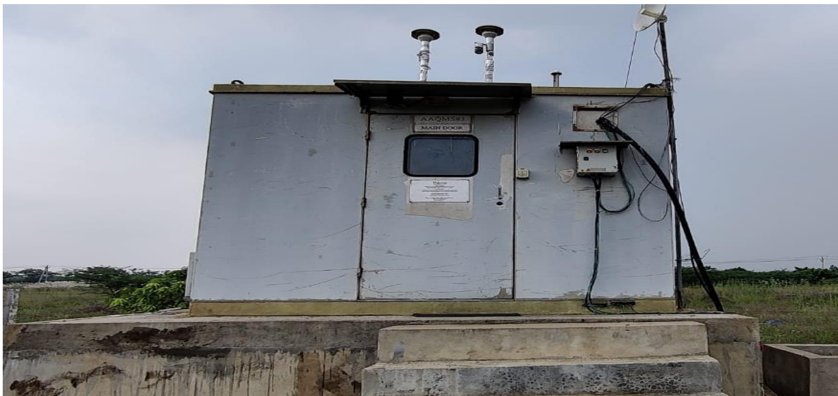
CONTINUOUS AMBIENT AIR QUALITY MONITORING STATION INSIDE THE PLANT
