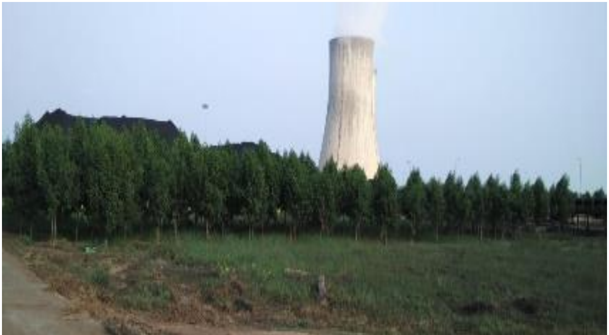
WIND BREAK PLANTATION AROUND COAL YARD
