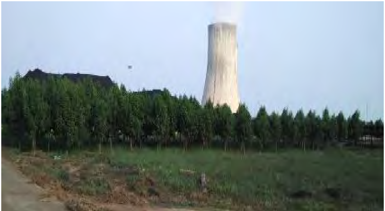
WIND BREAK PLANTATION AROUND COAL YARD
