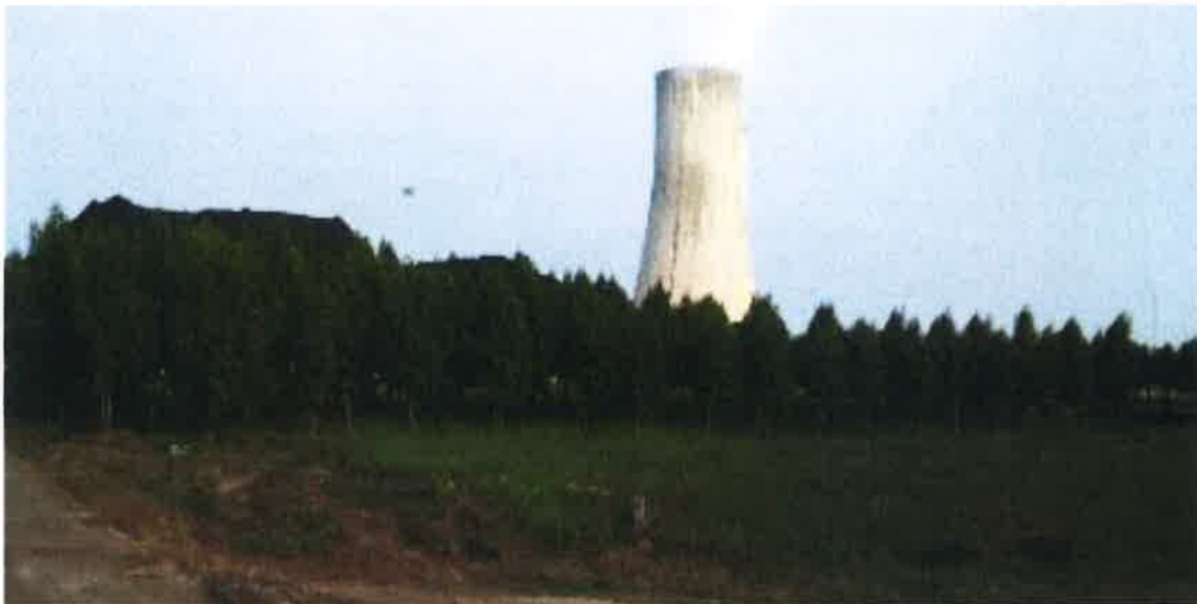
WIND BREAK PLANTATION AROUND COAL YARD
