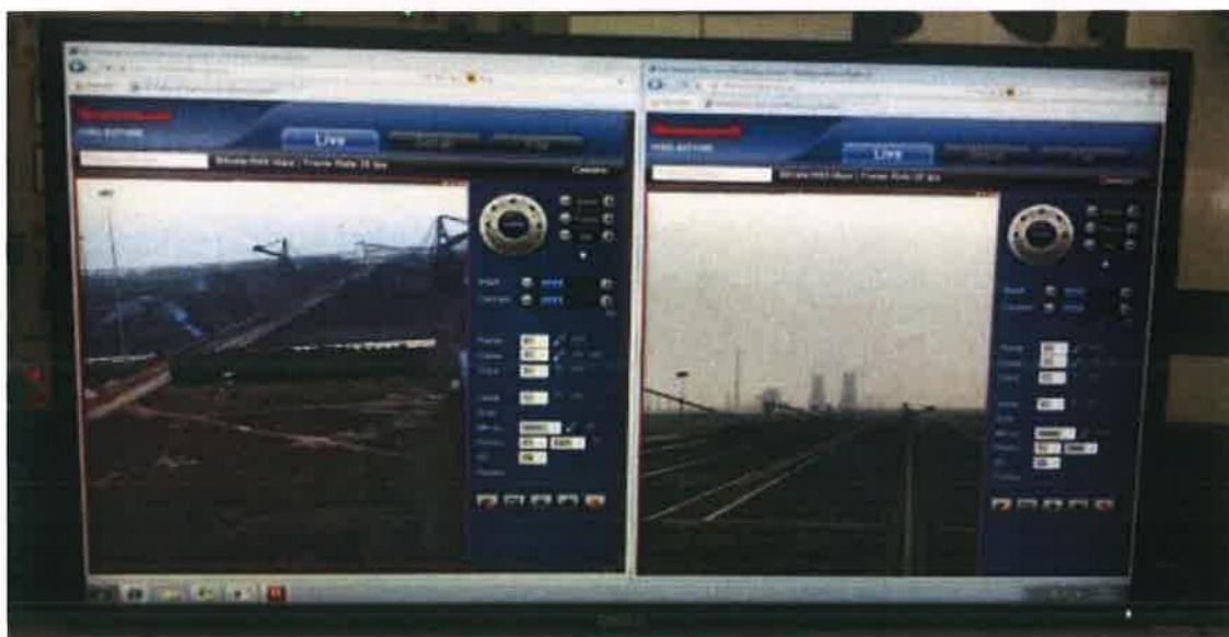
CONTINUOUS MONITORING OF DUST SUPPRESSION SYSTEM AT COAL YARD USING PTZ CAMERAS
