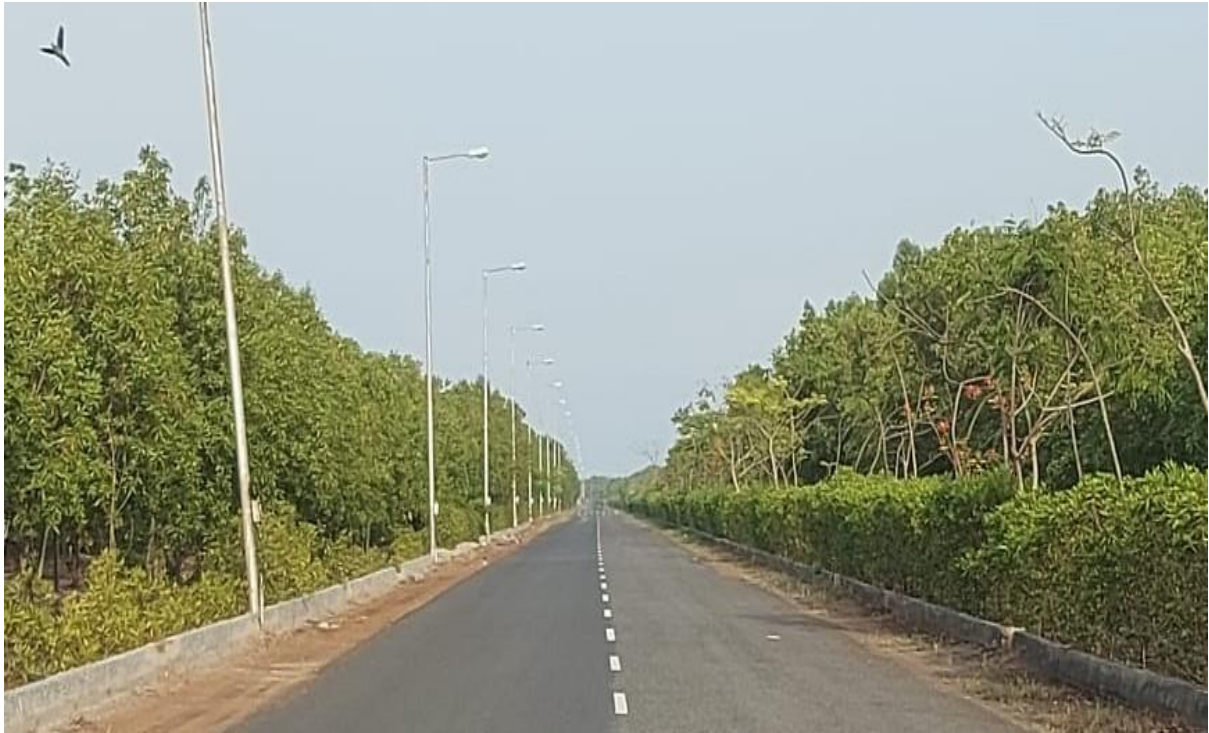
GREEN COVER ALONG PIPE RACK & INTERNAL ROADS
