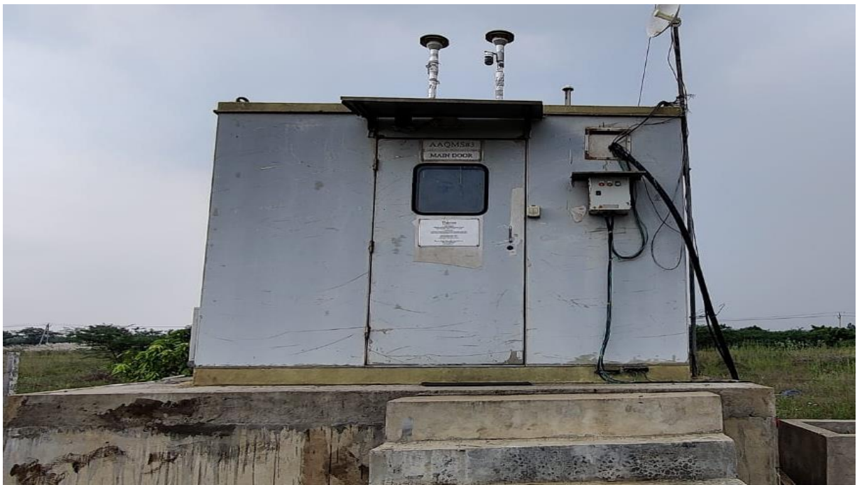
CONTINUOUS AMBIENT AIR QUALITY MONITORING STATION INSIDE THE PLANT
