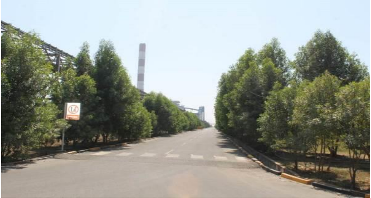
GREEN COVER ALONG PIPE RACK & INTERNAL ROADS
