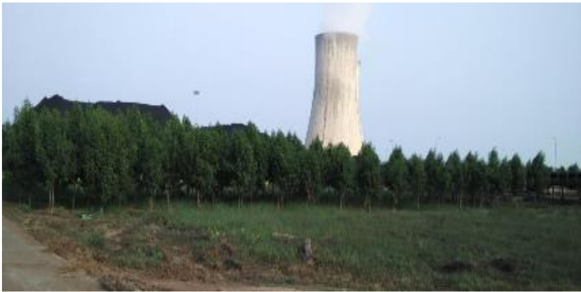
WIND BREAK PLANTATION AROUND COAL YARD
