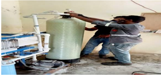
RO Plant Maintenance as part of CSR activity
