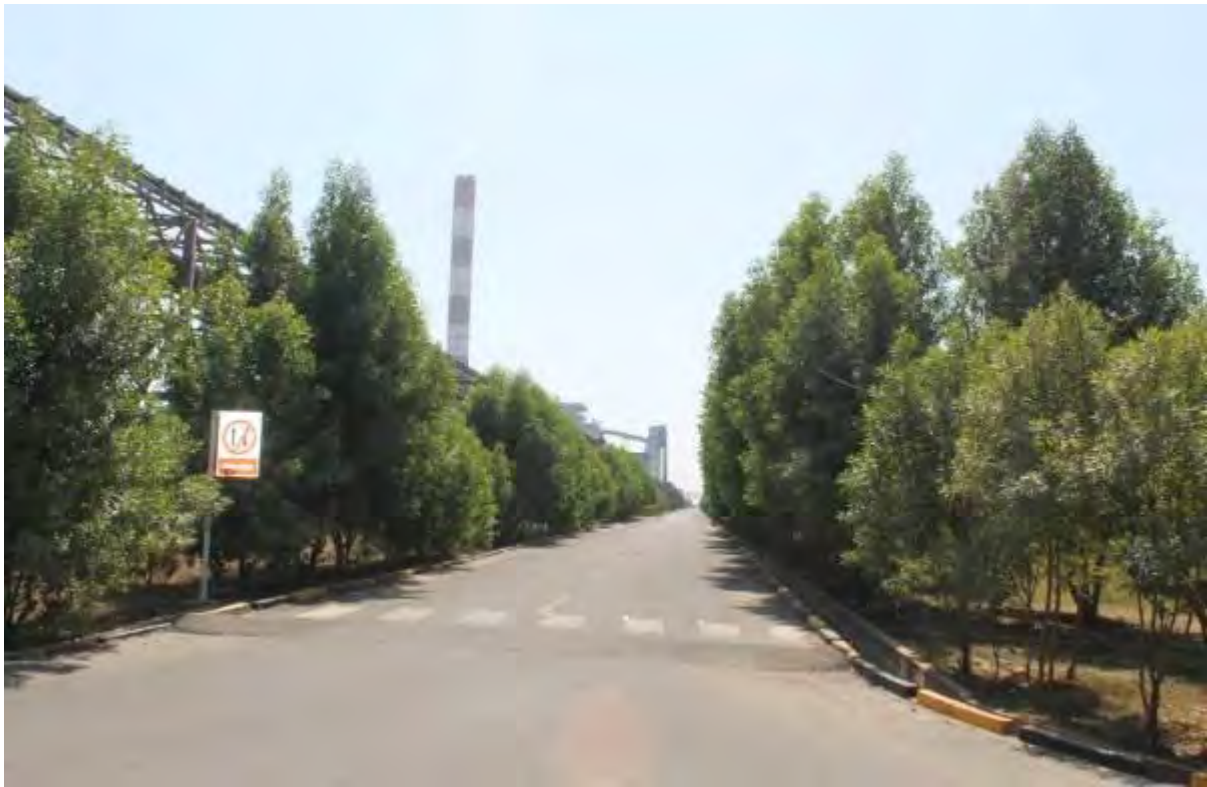
GREEN COVER ALONG PIPE RACK & INTERNAL ROADS
